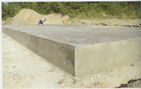
The completed slab awaits straw bales.
