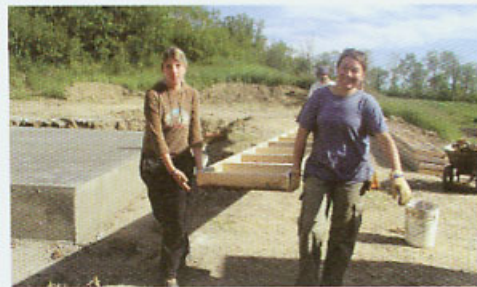
Formwork is removed from the completed frost-protected shallow foundation.
