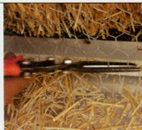
Trimming lath within the weep screed
