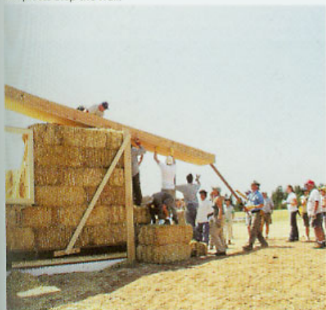
Short sections of an RBA may be raised at once if enough people are on hand. Notice the wall walkers ready to receive and place RBA pieces atop the wall.
