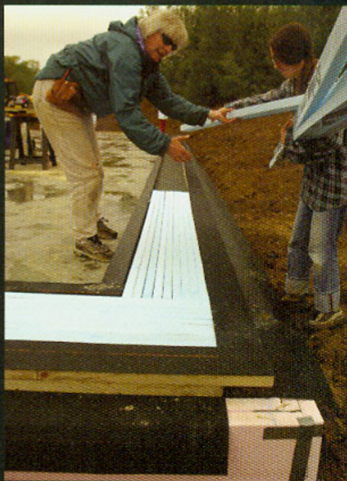
Detail of base plates with insulation
