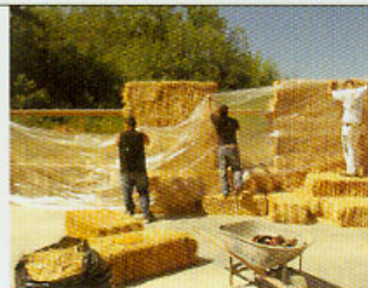
Tarps protect the bale wall from the elements.
