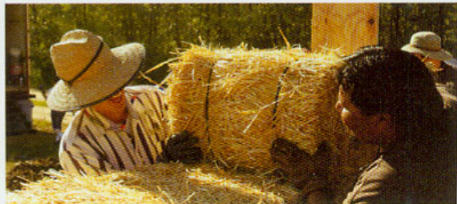
Half bales are often needed at window and door bucks.
