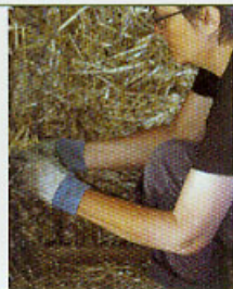
Use loose straw to fill the gaps.
