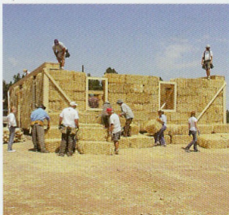
Build straw bale scaffolding along walls where RBA sections will be placed.
