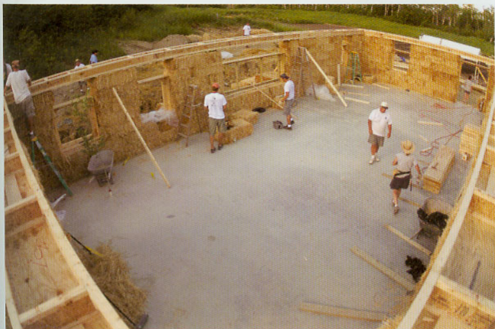
Short sections of an RBA may be raised at once if enough people are on hand. Notice the wall walkers ready to receive and place RBA pieces atop the wall.
