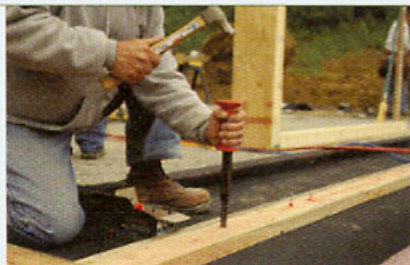
Powder-actuated fasteners hold the base plate to the slab.
