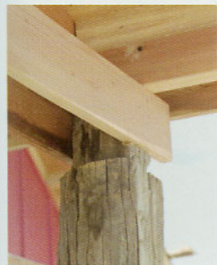
A salvaged post finds new life in a porch assembly.
